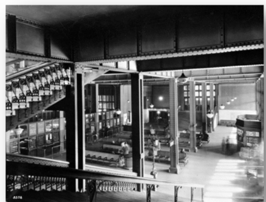
B & O's 24th and Chestnut Street Station's Lower Level, Waiting Room Looking East from Stairs, ca. 1920. Photograph. Library of Congress, Prints & Photographs Divisions, HABS PA, 51-PHILA, 405-15.
